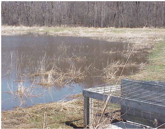
Basin and outlet trash rack
