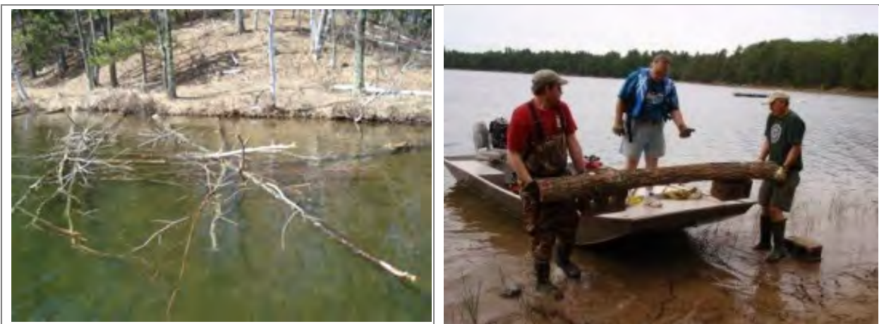
Photograph 8.4.6-3. Examples of fish sticks (left) and half-log habitat structures. (Photos by WDNR)
