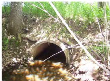
33- PRIVATE CULVERT MEADOWBROOK (RM 2.55)
