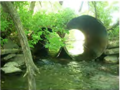
4- PRIVATE CULVERTS COCO CREEK (RM 0.81)
