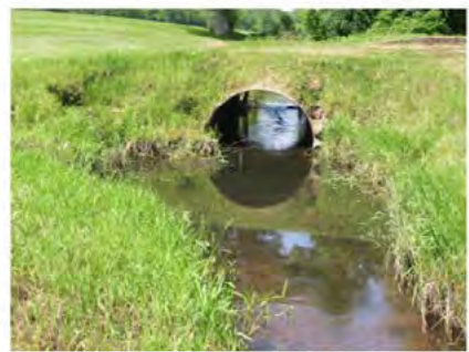
39- WESTERN LAKES GOLF CLUB CULVERT 3 ZION CREEK (RM 0.64)
