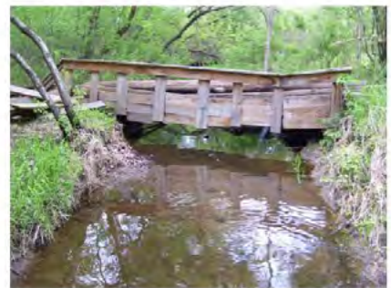
15-PRIVATE WALKING BRIDGE COCO CREEK (RM 3.54)
