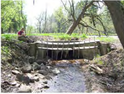
13- UNDERGROUND CULVERTS COCO CREEK (RM 2.94)
