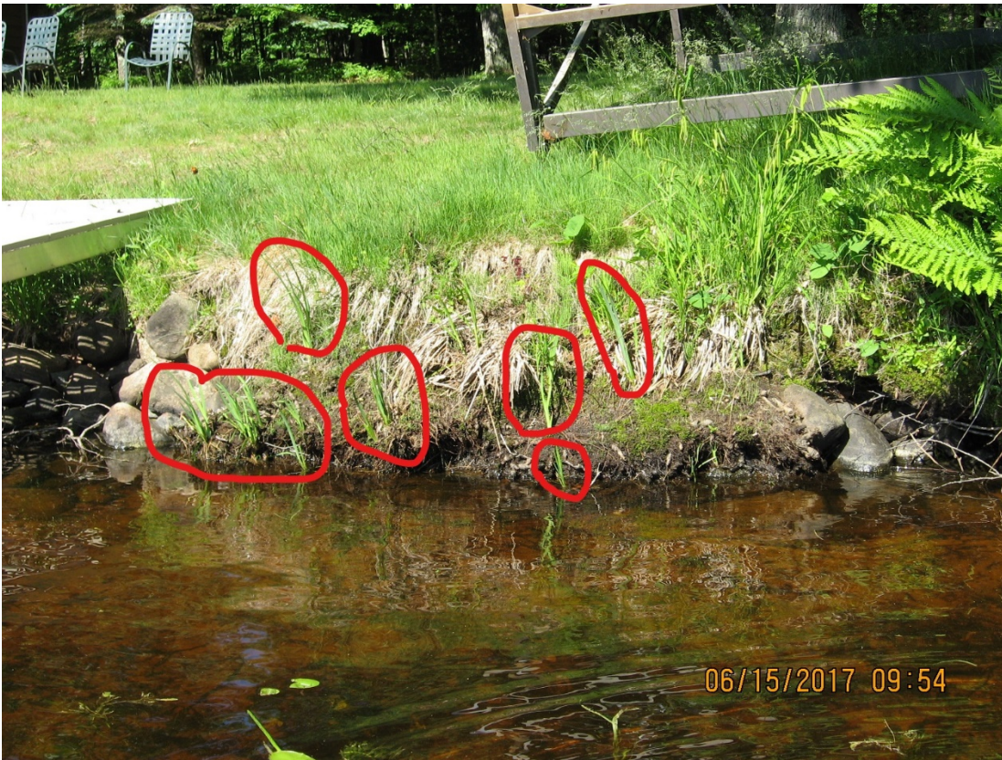
6/15/2017 Property 0200 dock north side "after" 9/8/2016 spraying. Some smaller YFI plants remain.
