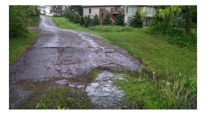
Runoff flows down entire landing driveway to the lake (5/23/16)  $(4,500 \text{ ft}^2 \text{ of hard surface} - \text{need } 937.5 \text{ ft3}$  of rock infiltration area to capture a 1" rain.)
