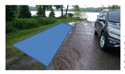
Install rock infiltration area under parking areas. Keep shallow to maintain separation to water table. East side installed in 2016. Top portion has sedimented in. Remove dirty rock and replace with clean.
