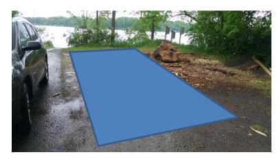
Rock infiltration – west side Rock size for both 1 1/2" clean, **level bottom,** rock across entire surface currently dirt.
