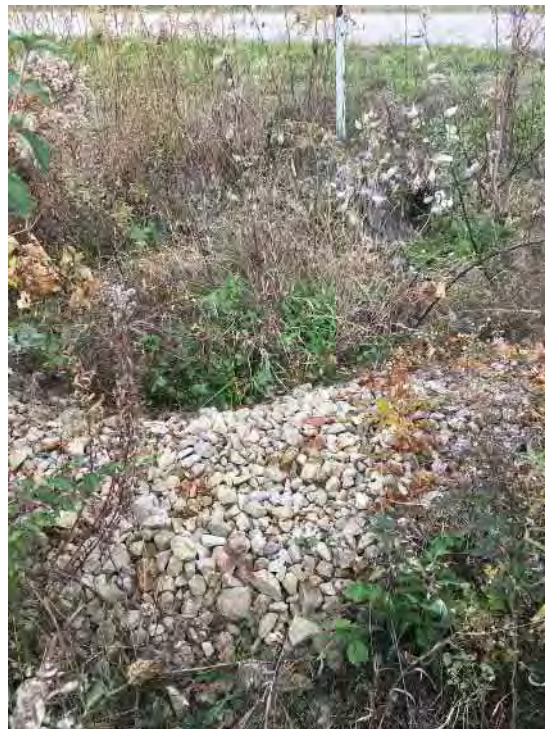
Shows rocks at culvert outlet in Velkommen Way
