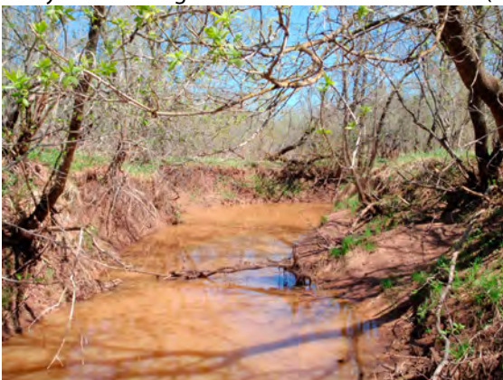
Erosion on Bluff Creek – unstable side slopes can not withstand erosive flashy runoff events
