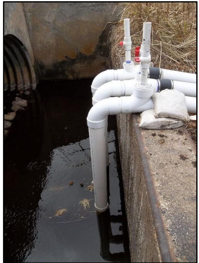
Figure 2. 6-inch siphons created using off-the-shelf plumbing supplies.
