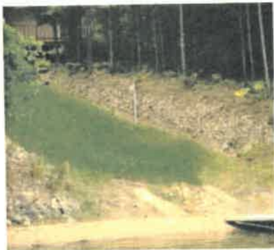
Lawn/Soil Sloping to Lake – the land slopes toward the lake and lacks natural vegetation that would prevent runoff/erosion (e.g., slope covered by lawn, bare soil, gravel, mulch)
