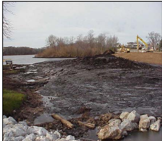
Figure 10. Picture of displaced lakebed sediment caused by the construction of the berm separating Silver Creek from the lake. Much of the displaced sediment was removed to allow access to the lake.
