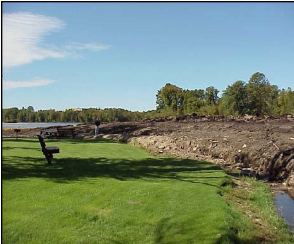
Figure 10. Picture of displaced lakebed sediment caused by the construction of the berm separating Silver Creek from the lake. Much of the displaced sediment was removed to allow access to the lake.
