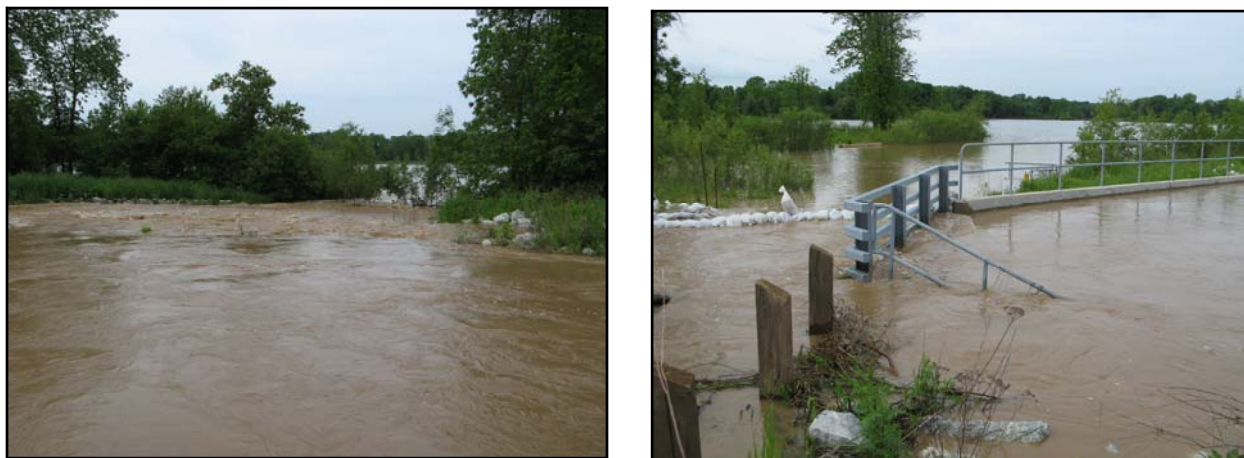
Figure 12. Pictures of Silver Creek overflowing the berm and entering Silver Lake in June 2008. The water level of the lake was raised over 3 feet during this time.
