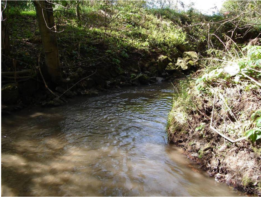
Figure E-3. Typical bank erosion along the outside of stream bend of Hardies Creek
