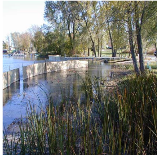
Picture 6. Emergent vegetation establishment at English Lake County Park following the first growing season.
