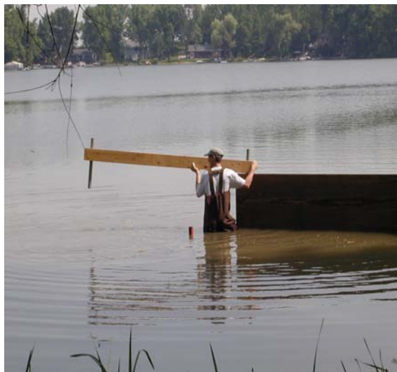
Picture 3. Wave break installation at the English Lake County Park.
