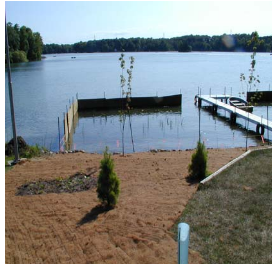
Picture 16. Wavebreaks and erosion blanket that were installed at the Pigeon Lake site.
