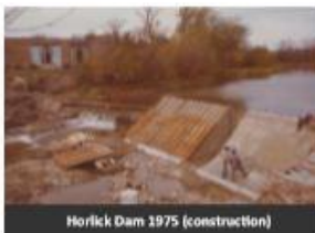
Horlick Dam 1975 (construction)
