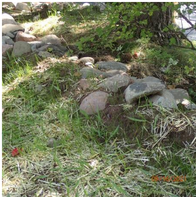
Photo 7: Sep 16, 2021. An earth and rock diversion was intalled.
