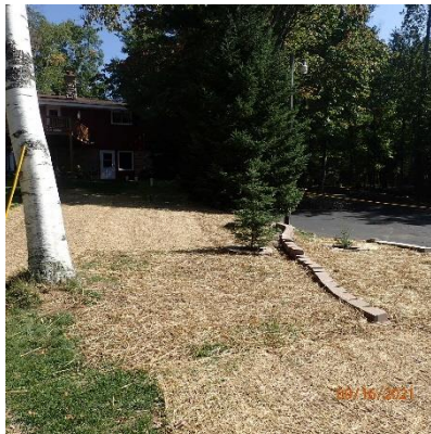
Photo 8: Sep 16, 2021. Straw mats and grass seed were installed to minimize erosion.
