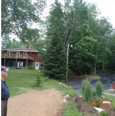
Photo 1: June 24, 2021. The Rogers property sheds water to the neighboring property.
