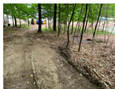
Photo 3: Diversion Path After June 2019
