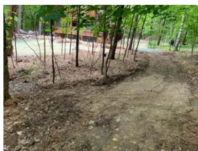
Photo 1: Diversion Path After June 2019
