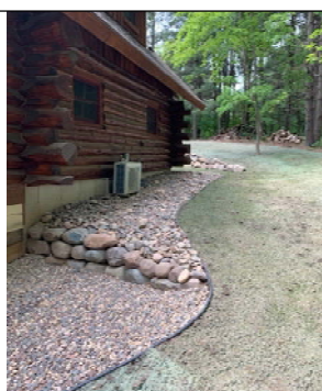
Photo 2: Infiltration Pit North Side After June 2019
