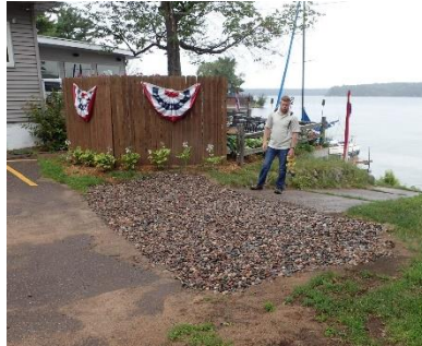
Figure 15. Impervious surfaces and straight trail/road access allow runoff to speed up and brings phosphorus laden sediments to the lake. This site (not on Pioneer Lake) was augmented with a water infiltration pit to minimize runoff going into the lake.
