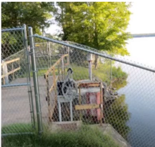
Photo 4 : Twin Falls Dam, 2017. PLA.
