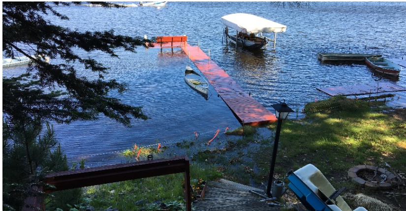
Photo 3: Flooding damage on one Pioneer Lake Property (2017). Mary Finlay.
