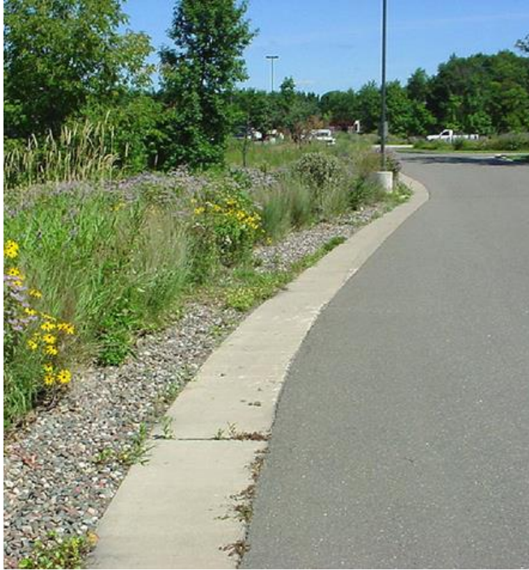
Figure 22: Infiltration Trench (MPCA)
