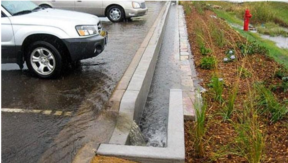
Figure 25: Level Spreader (MPCA)
