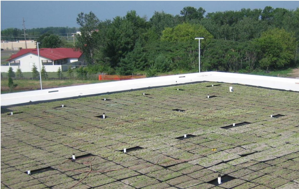
Figure 27: Green Roof on Amery Regional Hospital (EOR)
