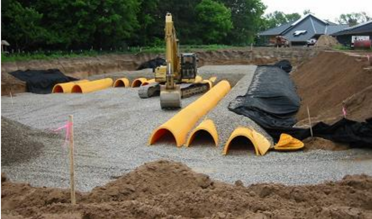
Figure 23: Underground infiltration chambers being installed under a parking lot (EOR)
