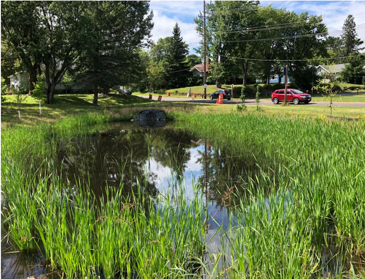
Figure 28: Stormwater Wetland in Cumberland (EOR)
