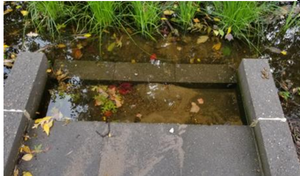
Custom Concrete Forebays
