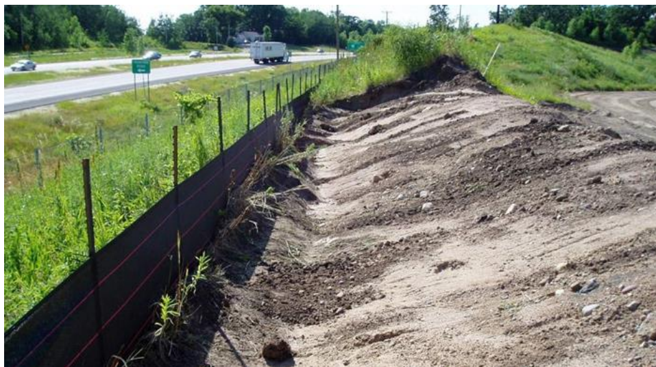
Figure 8: Installed silt fence will minimize sediment leaving a site and contaminating surface waters
