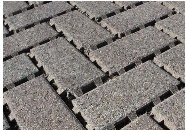
Figure 19: Permeable Concrete Pavers
