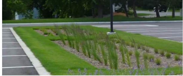
Figure 15: Vegetated Filter Strip
