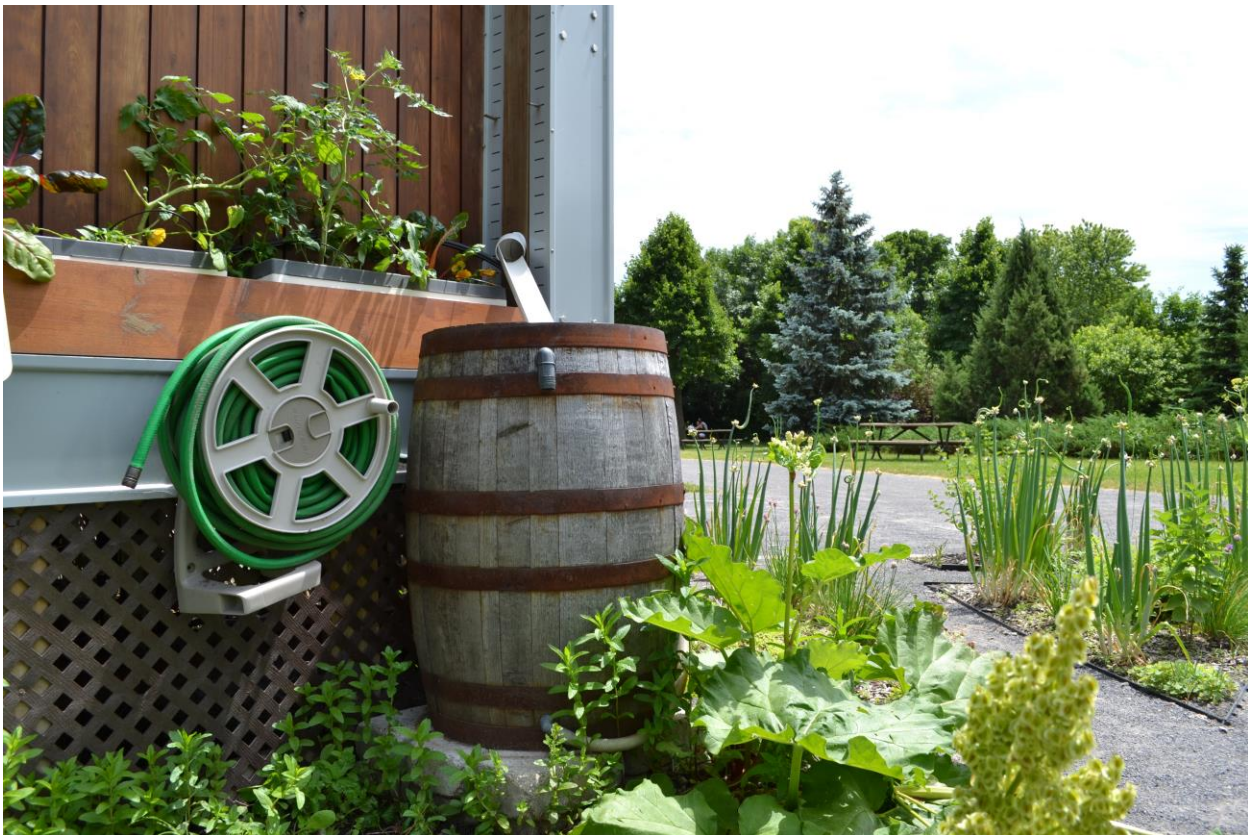
Figure 26: Rain barrel for harvesting roof runoff
