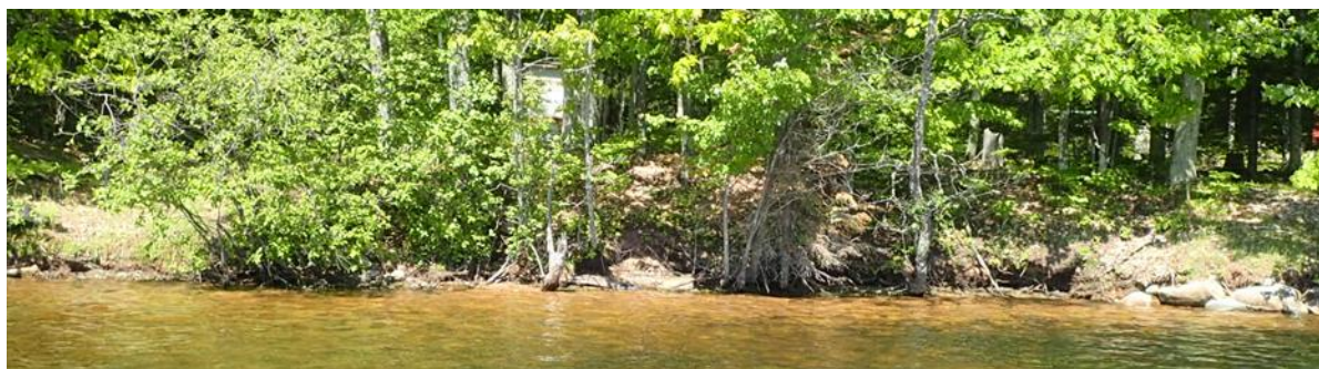
Figure 11. Bank erosion on Pioneer Lake likely caused by flank erosion from the adjacent riprapped area.
