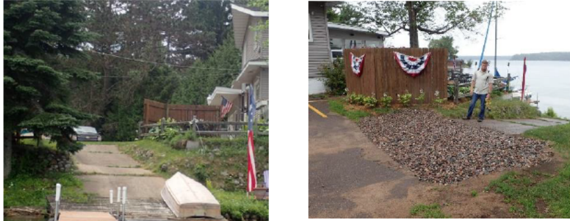
Figure 15. Impervious surfaces and straight trail/road access allow runoff to speed up and brings phosphorus laden sediments to the lake. This site (not on Pioneer Lake) was augmented with a water infiltration pit to minimize runoff going into the lake.
