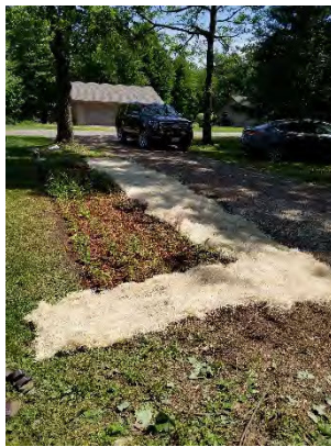
Photo 8: July 24, 2020 rain garden finished job
