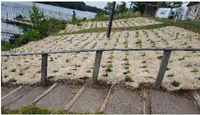
Photo 7: June 21, 2019 finished job
