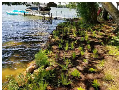
Photo 7: July 10, 2020 native planting finished job
