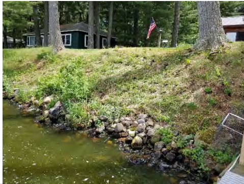
Photo 8: June 18, 2022 finished job
