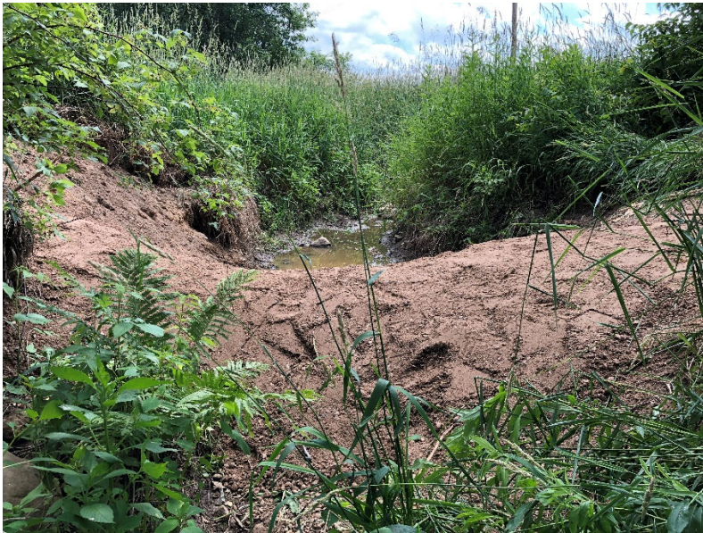
Compacted swale in place, 3' high by 10' long and 15' wide
