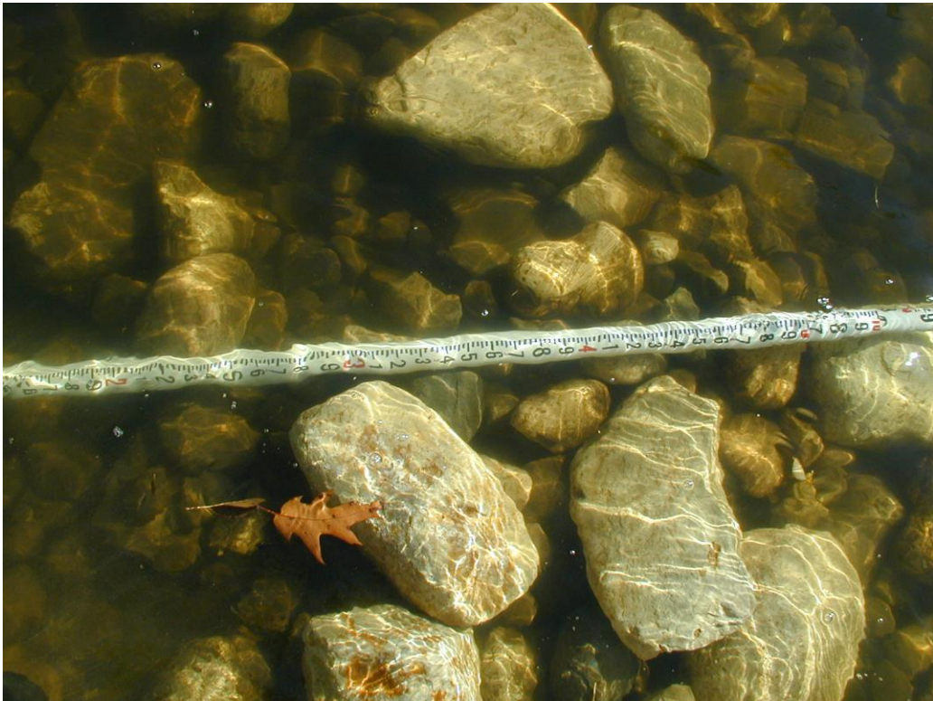
Photo 10. Typical reef substrate mixture of (2-in to 5-in and 6-in to 12-in dia. alluvial stone) constructed in moderate-shear stress and velocity areas. Approximately 20% of shoal area (0.10 acre).
