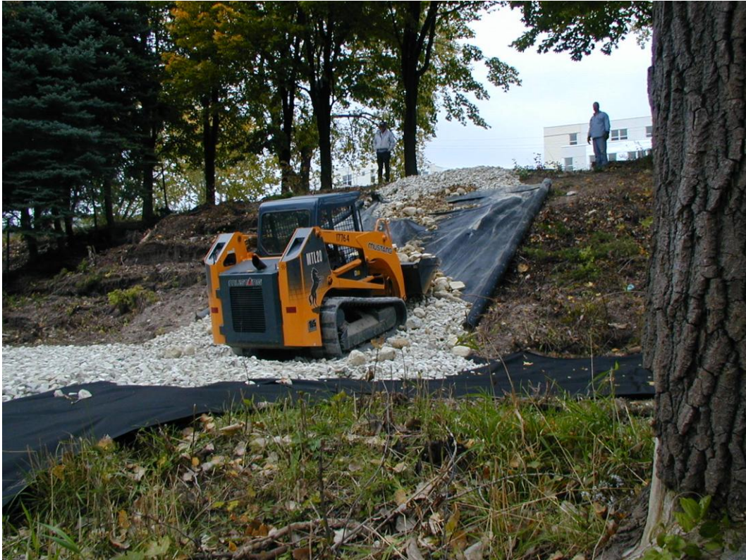
Photo 1. Construction of haul road to waters edge and future temporary causeway.
