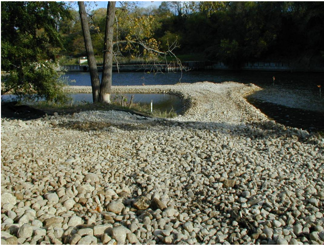
Photo 4. Looking northeast along haul road and temporary causeway. Note quality of stone generally clear of fines and the increase in thickness of stone for causeway to avoid equipment contact with river.
