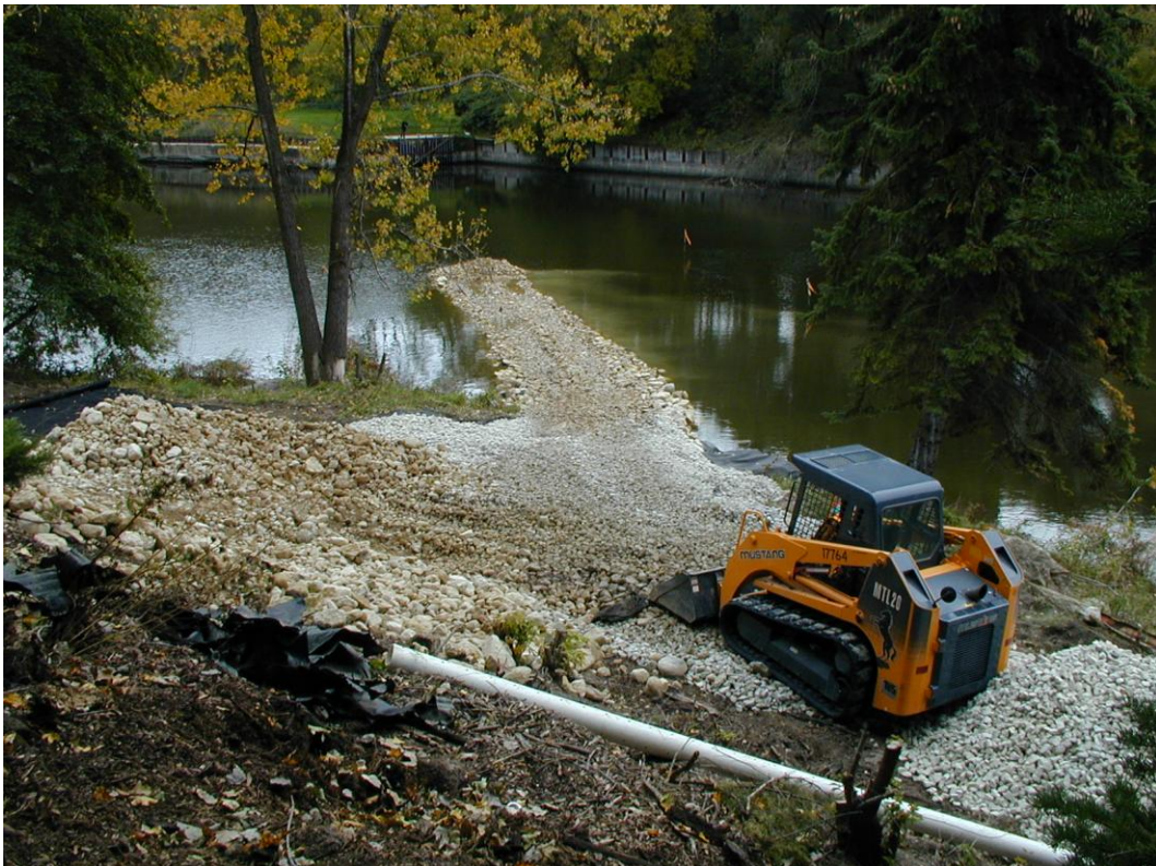
Photo 2. Looking northeast along haul road and initial leg of temporary causeway.
