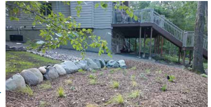
One of Gartland's rain gardens
