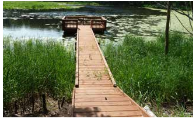
Observation platform - NE Pond Preserve
