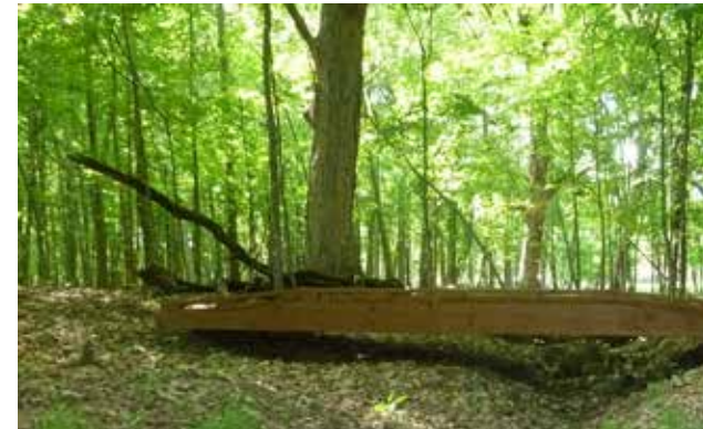
New bridge - Johnson Preserve
