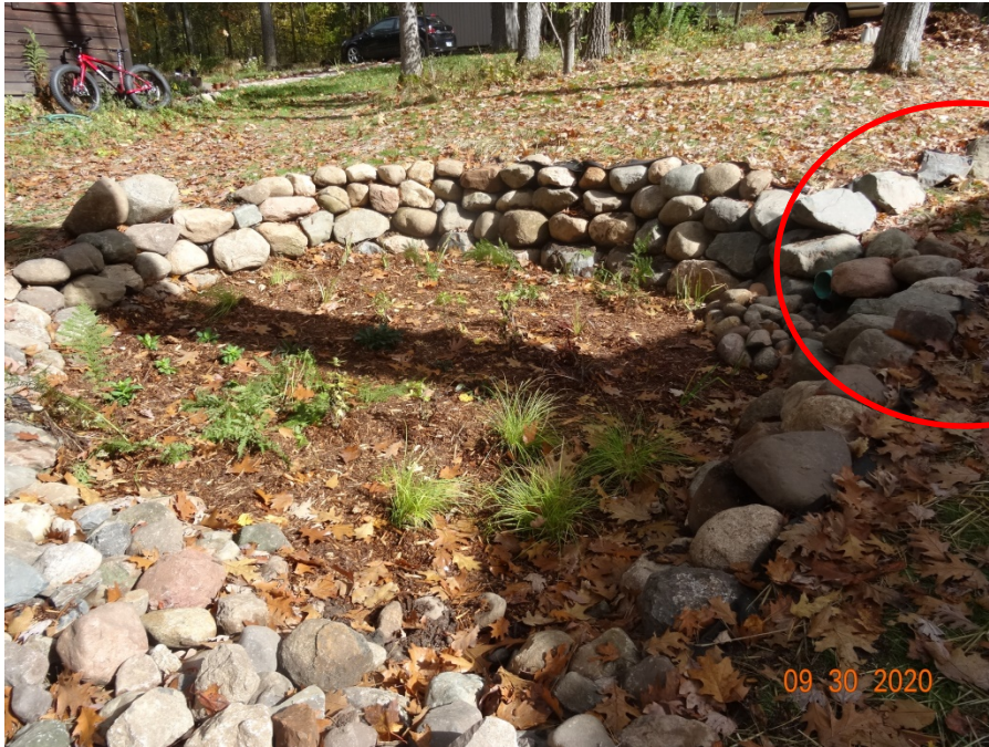
Rieke Before: September 30, 2021 Grassed inflow eroded with storm events – off photo
