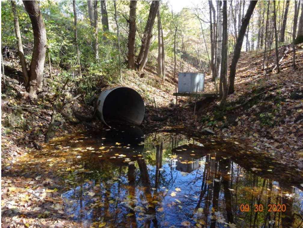
DLC Rock Creek Culvert
