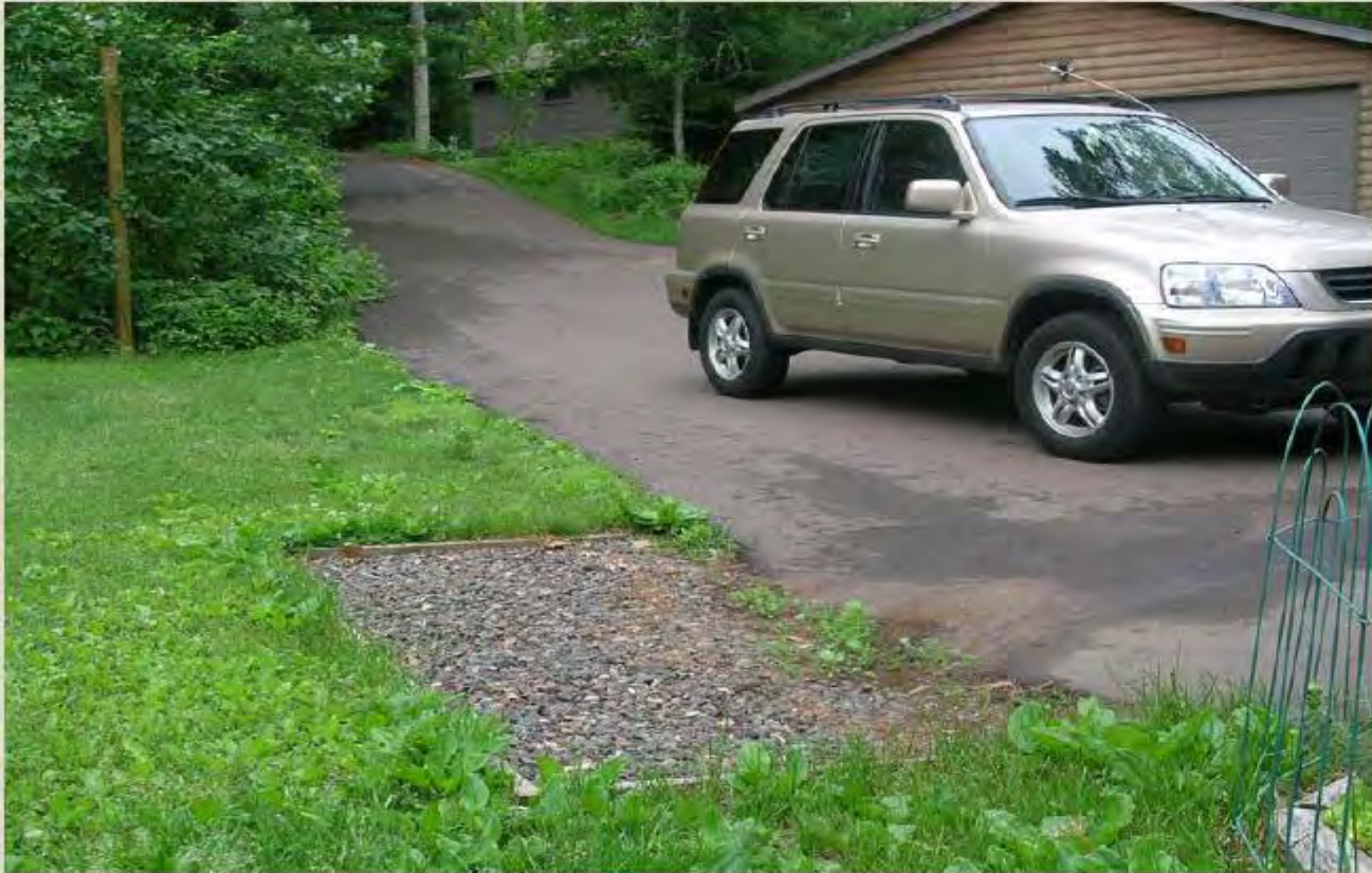
Rock Infiltration Pit
