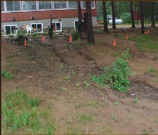
Erosion from bare soil
