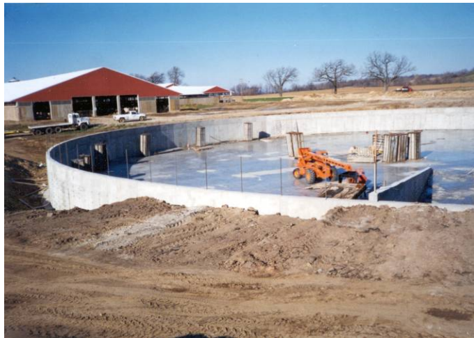
Construction of a concrete manure storage facility at a CAFO
