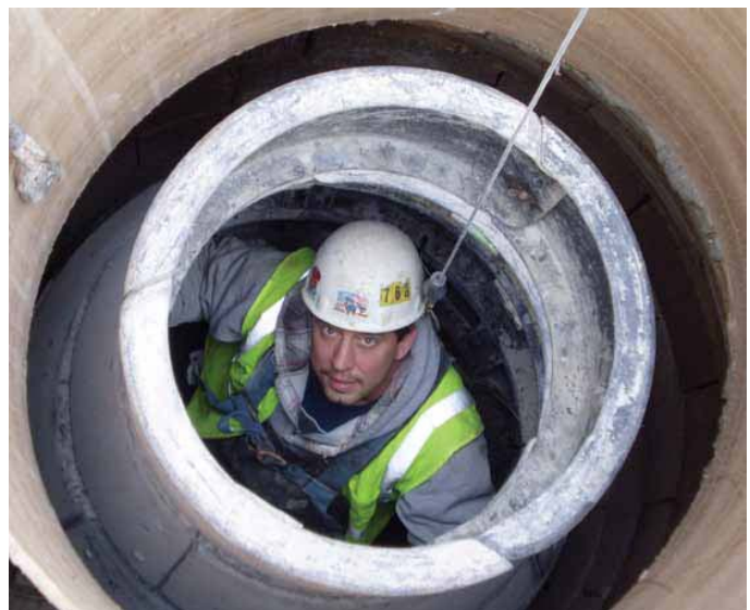
Reconstruction of an old manhole in Stevens Point, WI.
