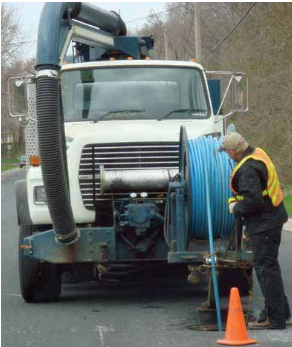
Cleaning out a sewer in Stoughton, WI.
