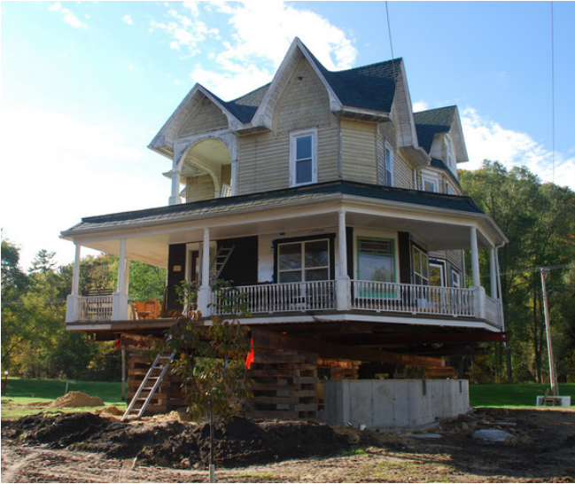
A Victorian home in Soldier's Grove, WI being elevated to protect it from flood events (Fall, 2008).
