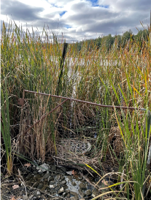
Photo 6. Dam structure outlet on unnamed impoundment looking upstream into unnamed impoundment.
