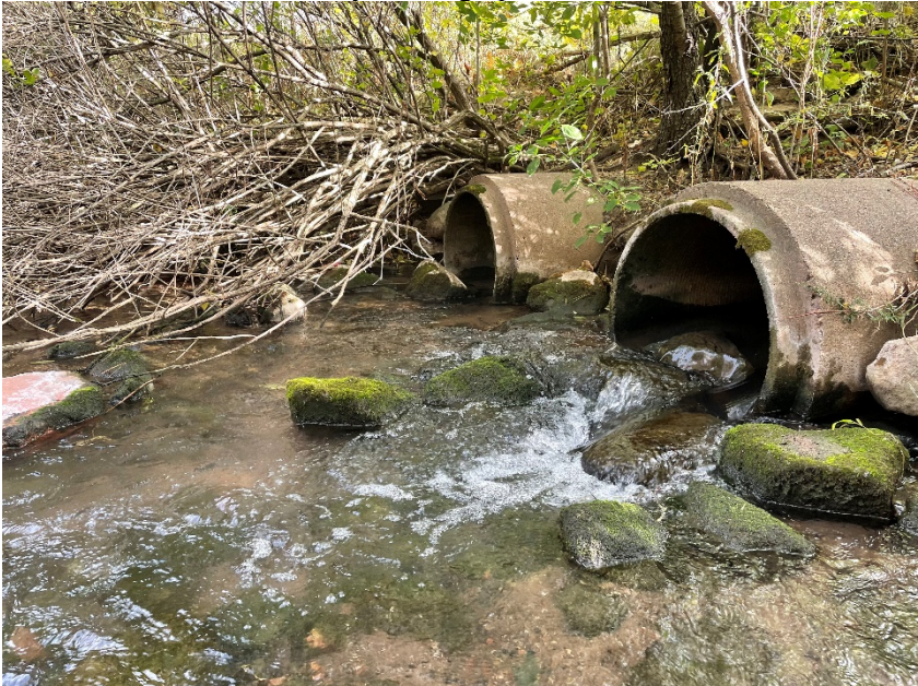
Photo 3. Unnamed tributary looking upstream at culverts at 7 th Street Northwest.
