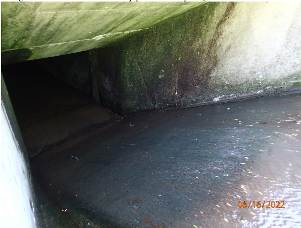
Site # 6 Downstream of Maribel WWTF at Unnamed Tributary (WBIC 3000159) east of I43 onramp, facing east. Culvert with 8-10 ft drop prevents fish passage.
