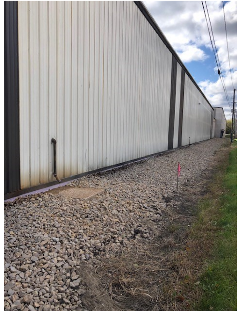
Drainage Ditch – South
