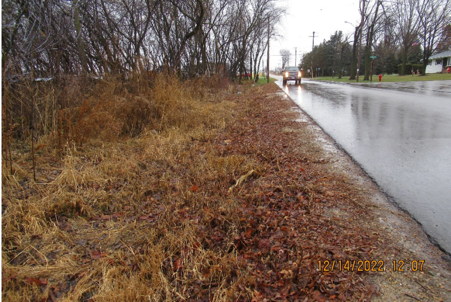
Bermed Drainage Ditch South of Flanagan Ave. – West
