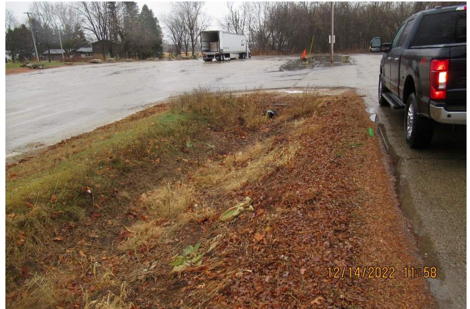
Drainage Ditch at SW Corner of Facility Property
