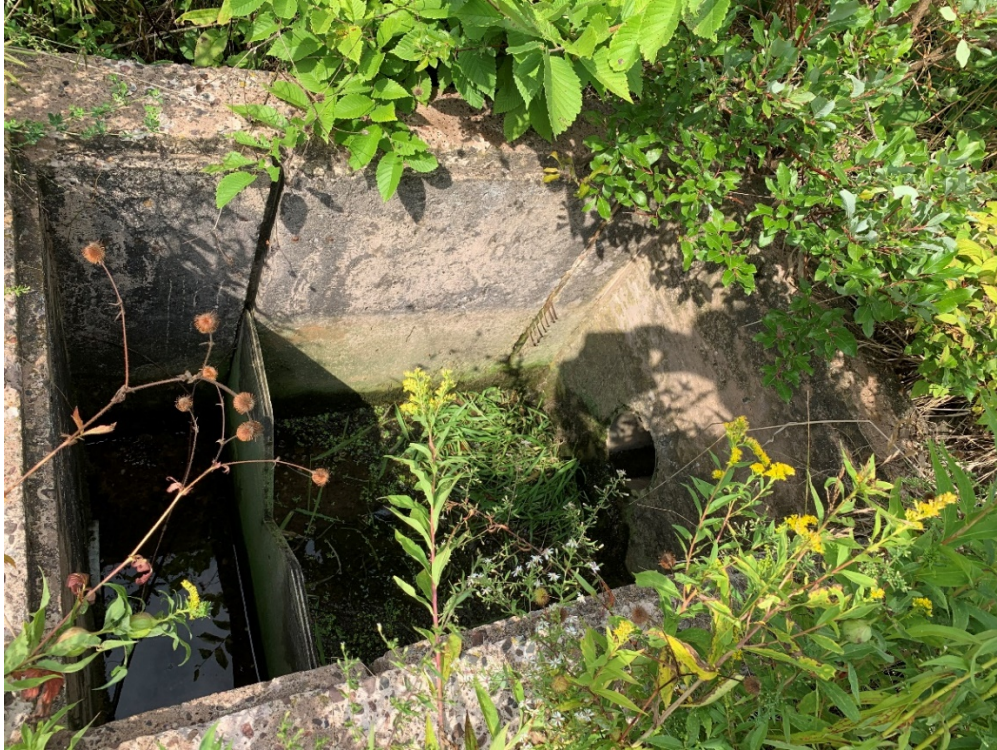
Site Photo 2. Concrete Structure with notched weir used to measure flows from ponds during discharge. Note the nails in a track center right of photo. Flows adjusted until water level reaches 2 nd nail from top during discharge.
