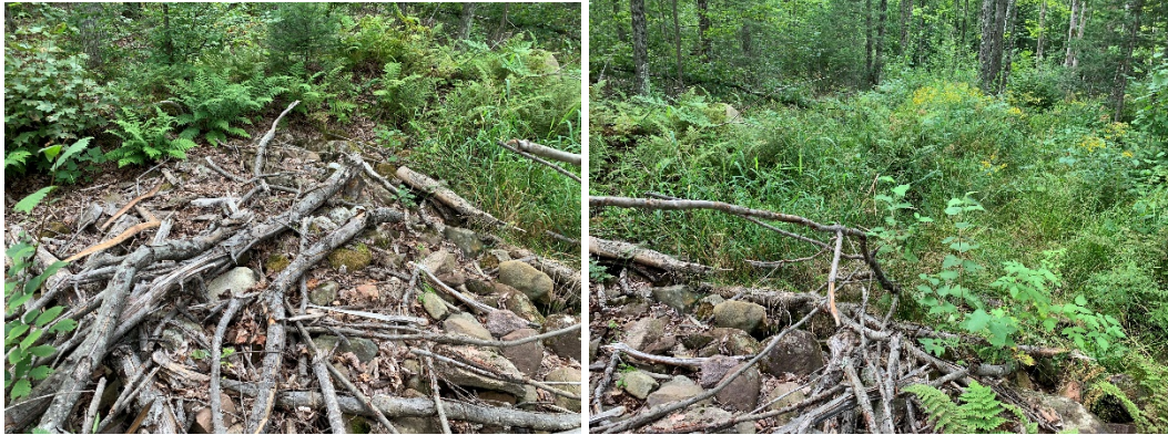
Site Photo 4. Pipe outlet coved by rocks and timber slash.
