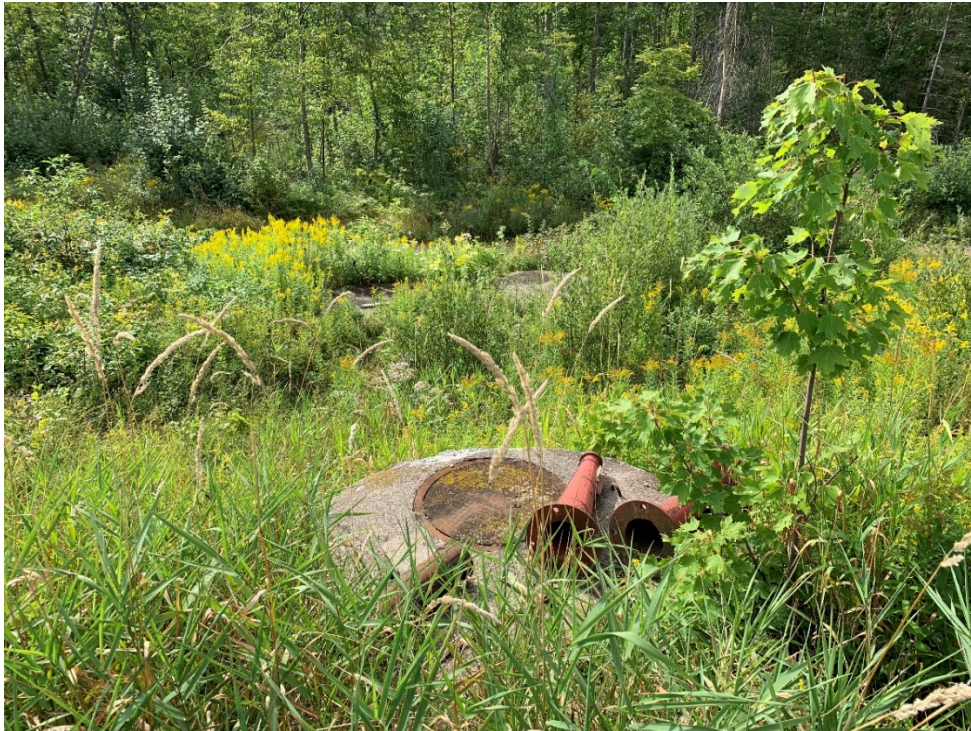
Site Photo 3. One of two concrete tanks observed between treatment pond outlet and discharge point.
