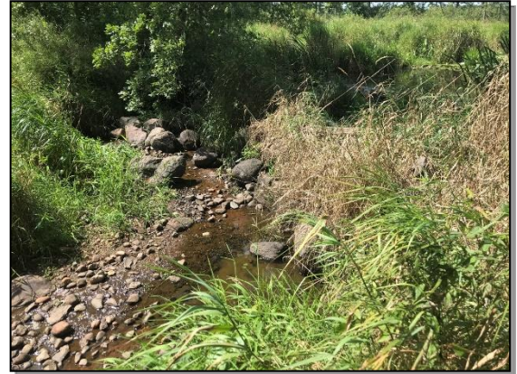
Staples Lake Dam
