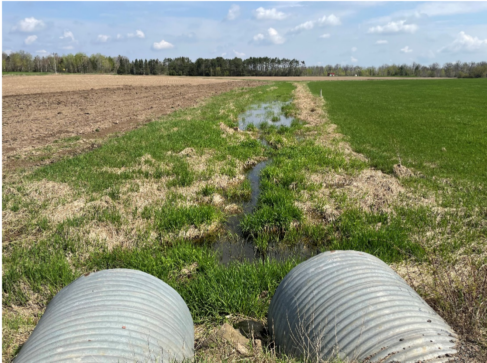
Photo 1. Unnamed Tributary at 18 ¼ Avenue looking upstream at survey area.
