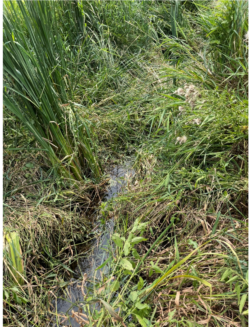
Photo 6. Channel through the wetland was covered by vegetation and difficult to find. Mucky bottom. (Here, vegetation has been trampled down to access it.)
