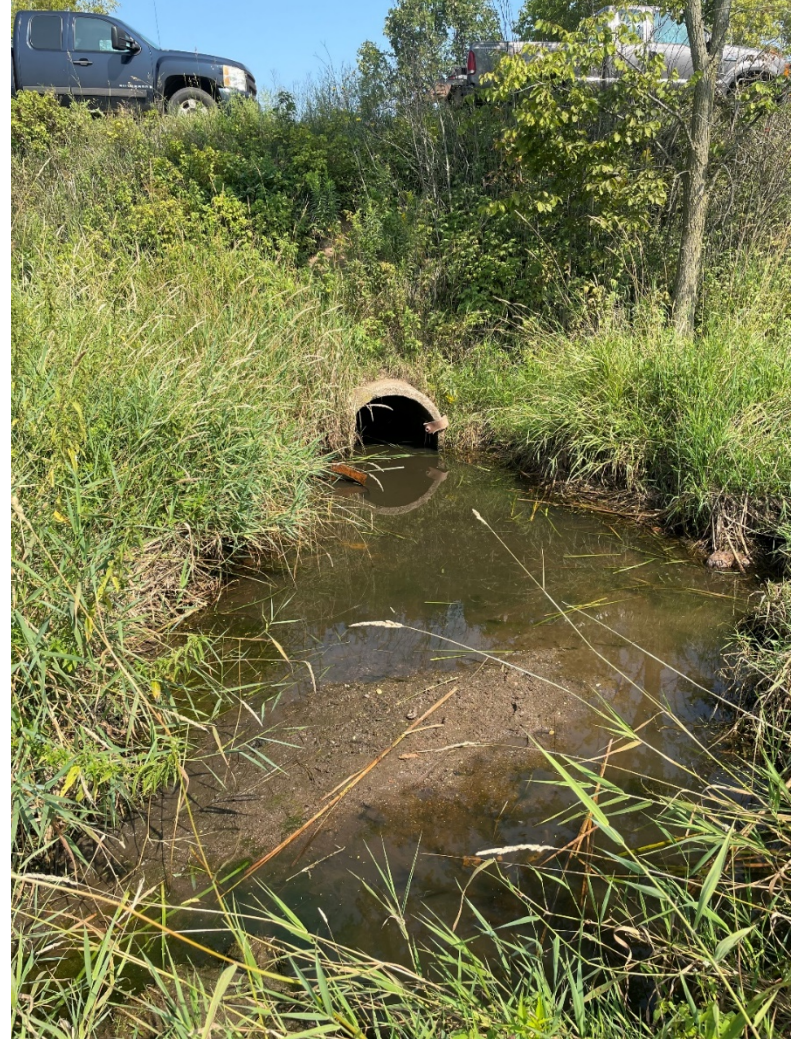
Photo 6. Upstream view of stormwater culvert pool.
