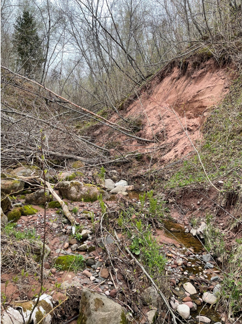
Photo 7. "Main channel" bank erosion downstream of Highway 13 looking upstream.
