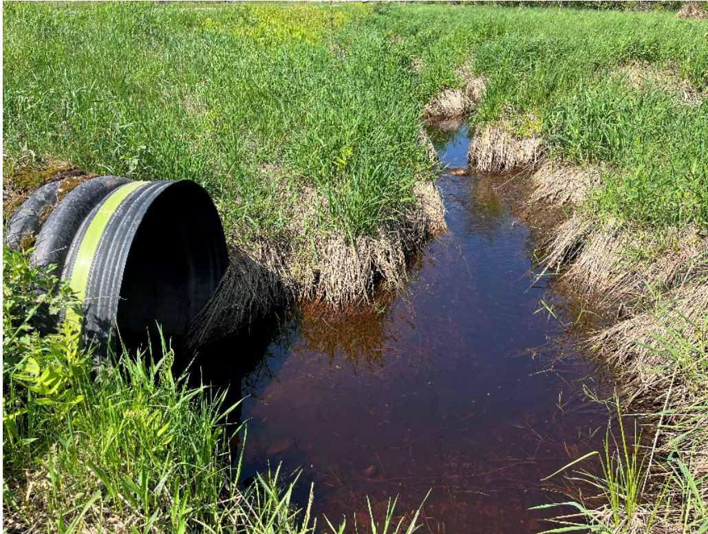
Photo 1. Unnamed tributary looking upstream (West) at culvert crossing on Townline Road.
