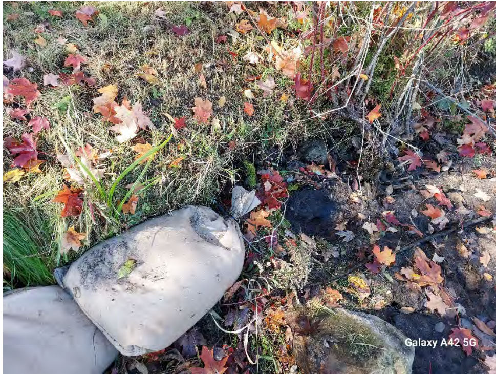
Photo 3: First course of bags being placed
