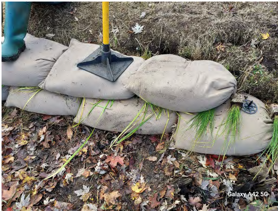
Photo 4: Second course of bags being placed, connector stakes placed (2 per bag) and roughly 3 plants per bag used.
