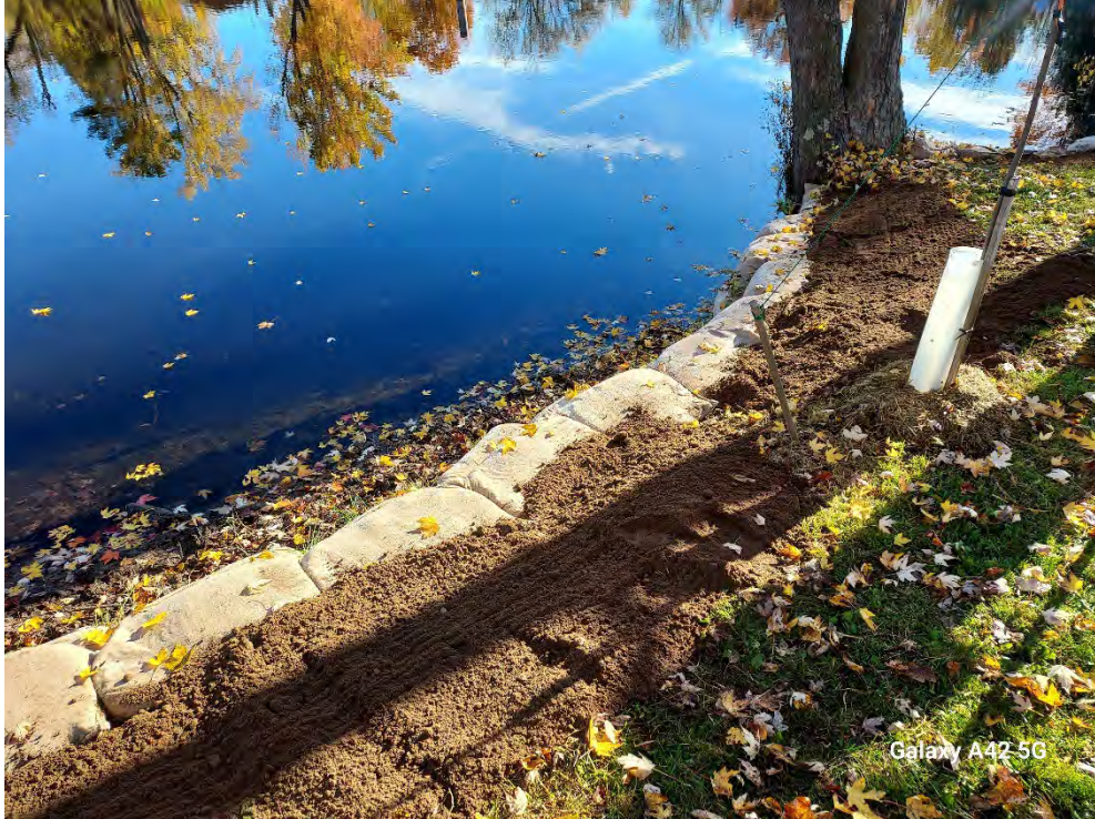
Photo 7: Backfilling behind bags, allows for free drainage of water
