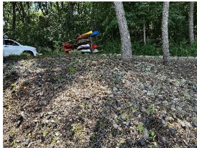
Photo 4: June 2024; Native shoreline area 1 during planting activities
