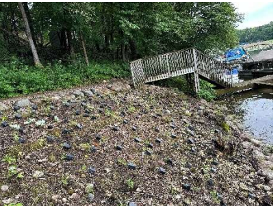
Photo 6: June 2024; Native shoreline area 3 during planting activities
