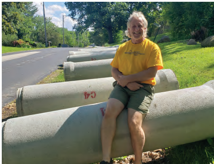
Jimmy DeGidio, checking out the materials that will be used for the Park Road reconstruction.
