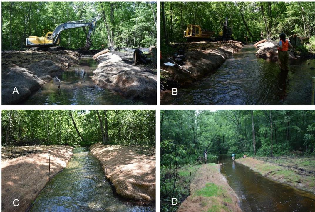
Fig. 2. Supporting Information. Photographs of diversion channel during construction (A,B) and when complete (C, D). The photographs in C and D were taken at baseflow and after a storm event, respectively.
