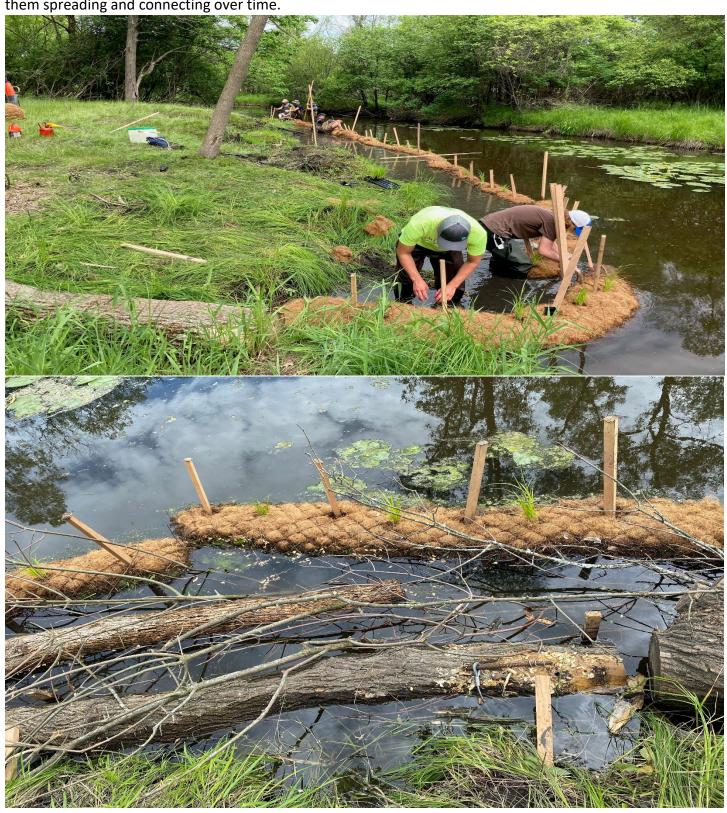
Hardwood was placed behind the logs and "duck billed" anchored in place.
