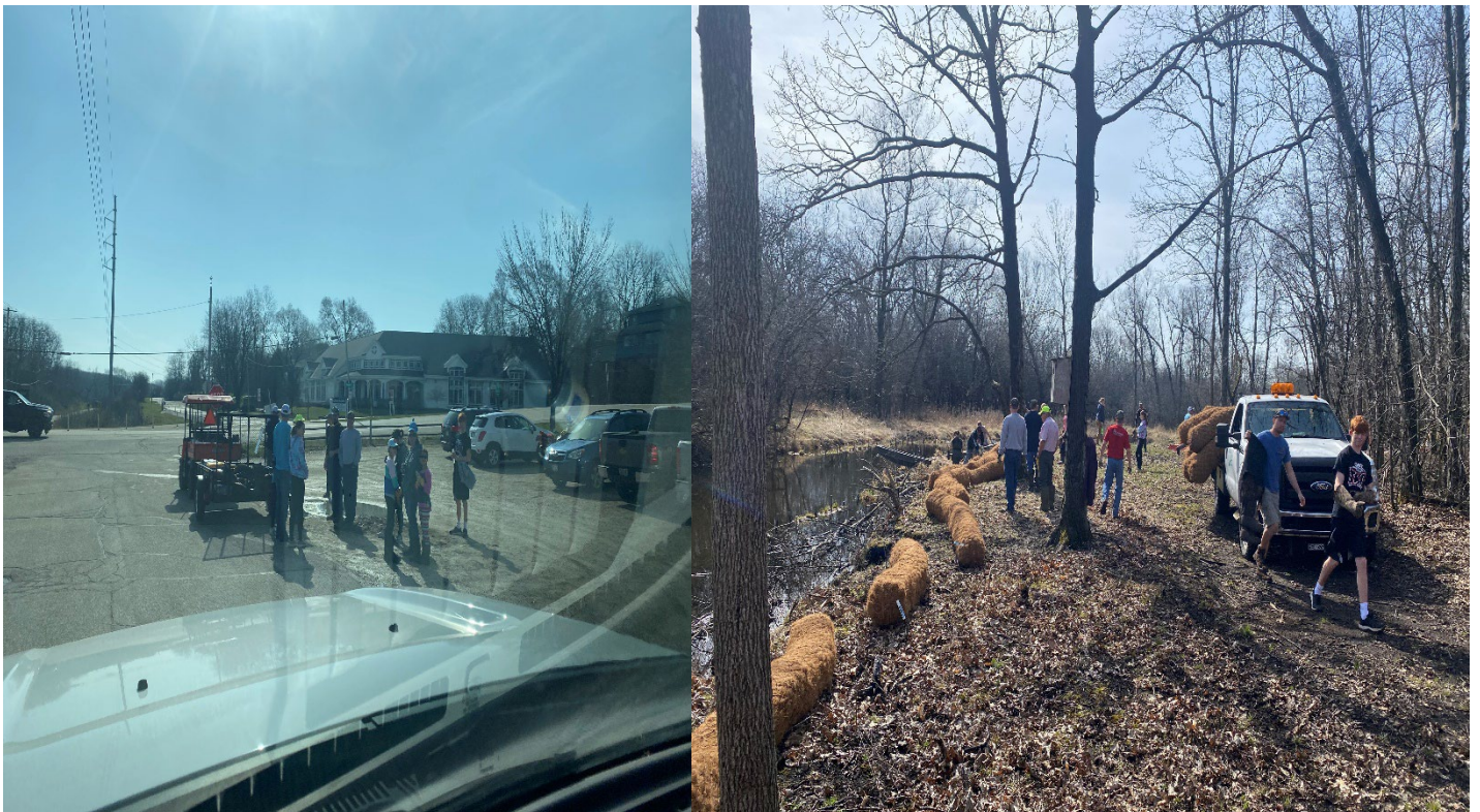
Loading up and staging the materials for placement.
