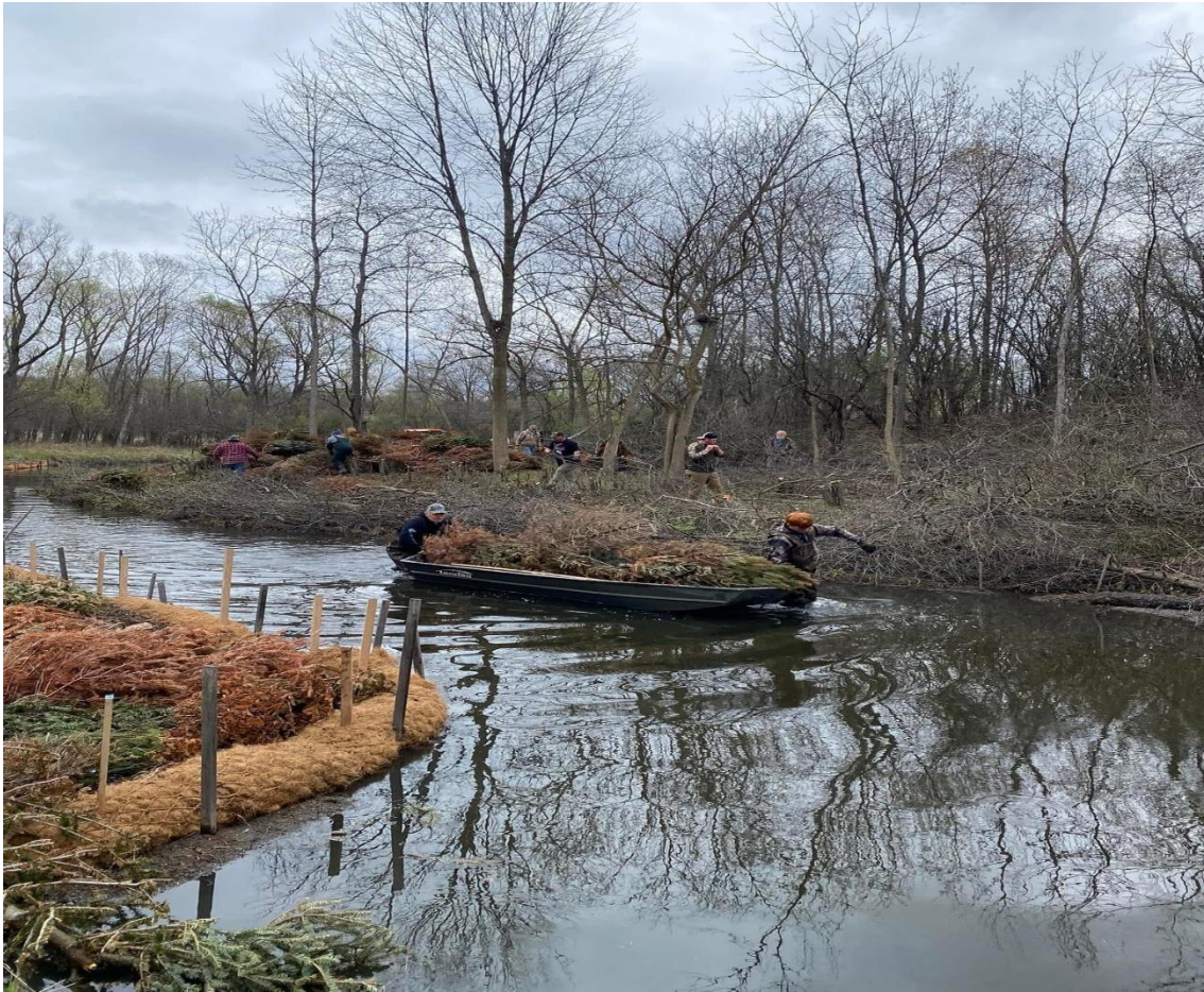
Figure 3: Greg and Levi Koepp hauling recycled Christmas trees to be used behind the choir logs. An example of a completed section of choir logs back filled with trees is seen on the left side of the image.
