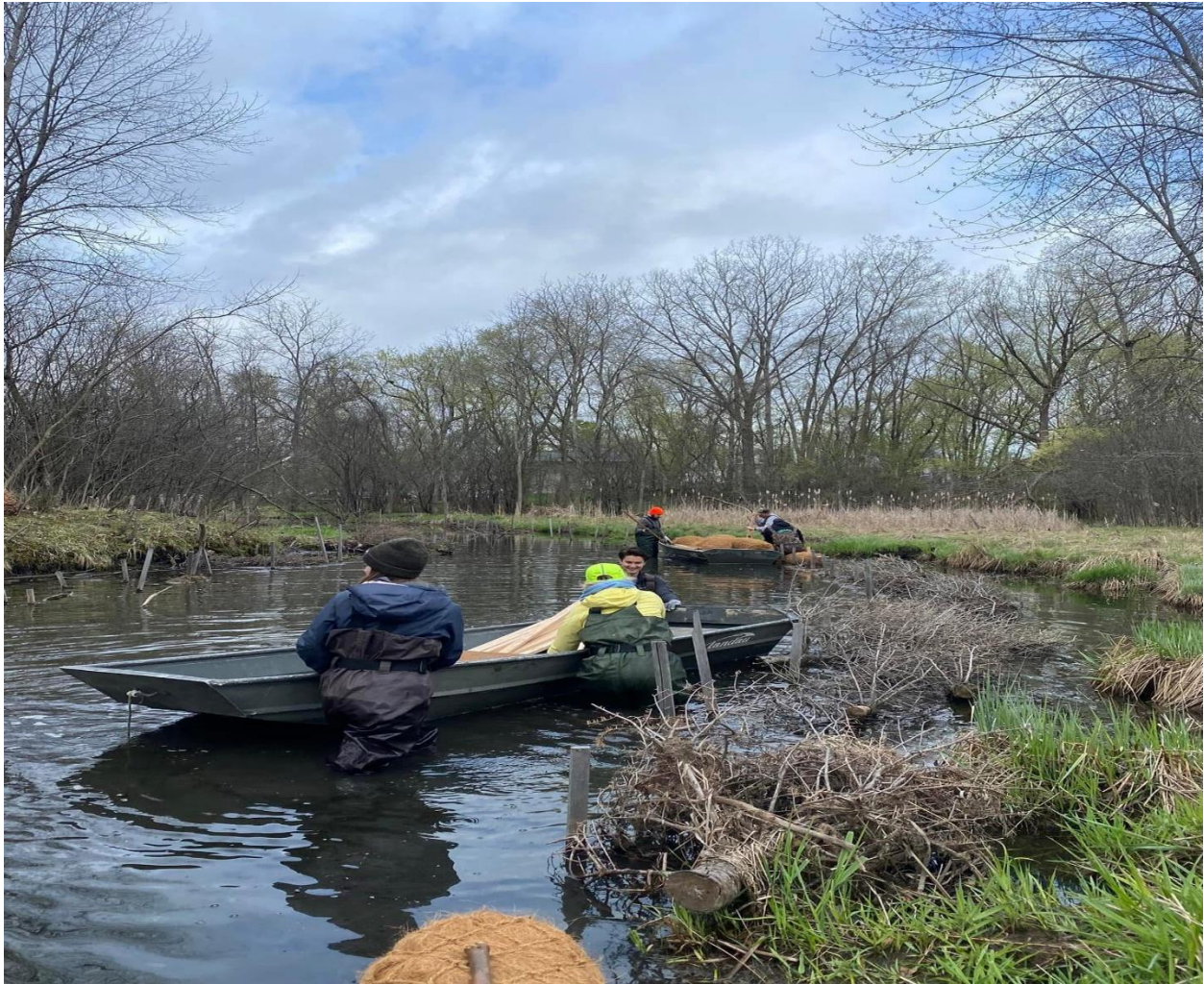
Figure 2: Volunteers using boats to haul choir logs and wooden stakes up and down the river.
