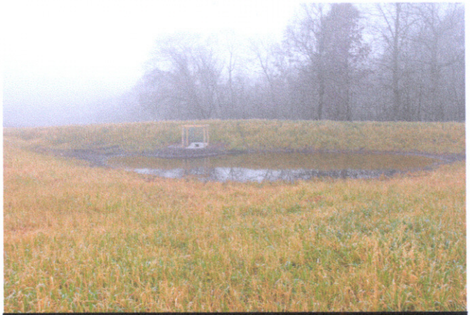
Completed grade stabilization structure.
