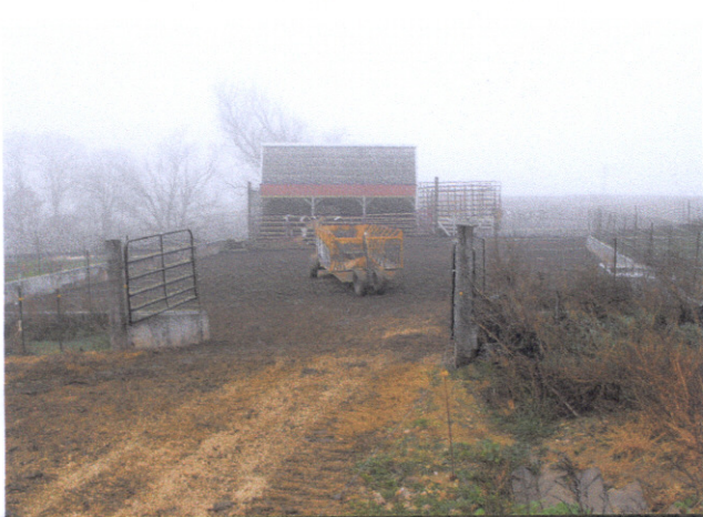
Completed barnyard system.
