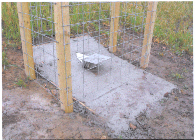
Inlet to pipe with trash rack.
