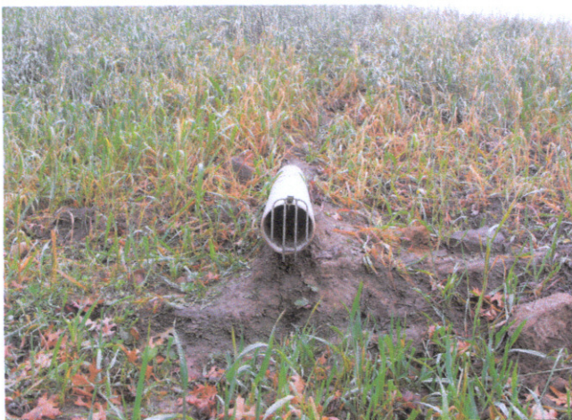
Outlet pipe with animal guard.
