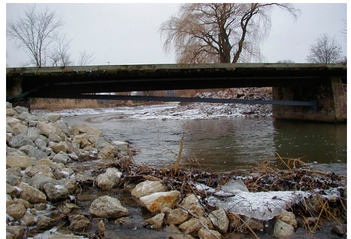
After Restoration, Kenosha County Club Dam
