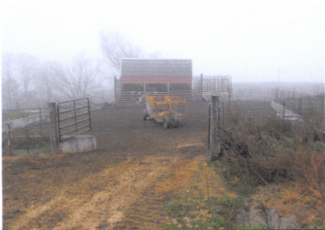
Completed barnyard system.
