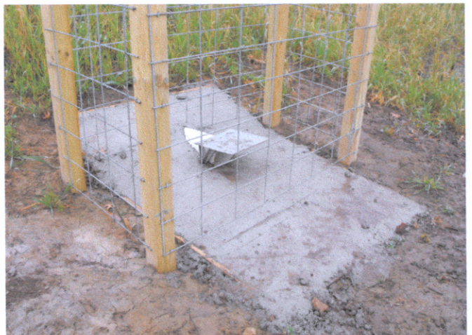
Inlet to pipe with trash rack.
