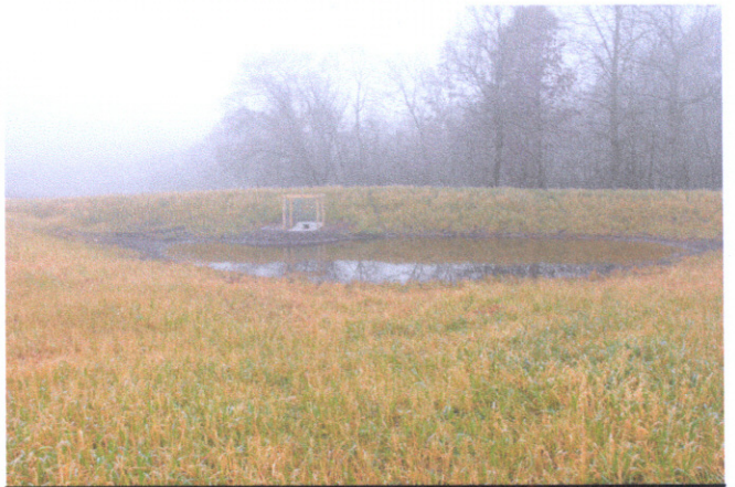
Completed grade stabilization structure.
