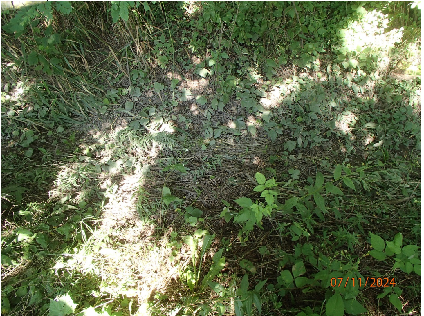
Photo 4: Surface ditch above storm sewer with indications of overflow, sediment deposits. Photo taken by David Bolha on July 11 th , 2024.
