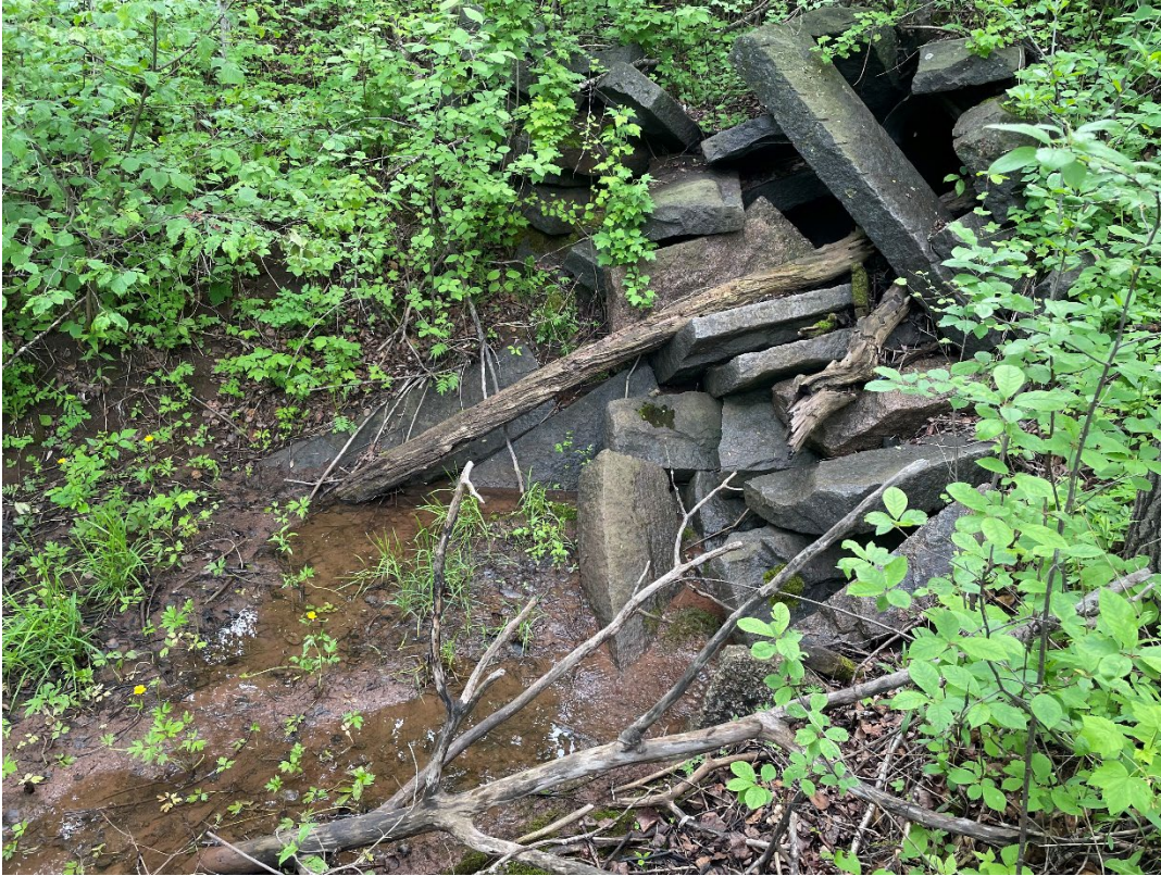
Photo 1. Unnamed Tributary culvert downstream of 39 th Avenue (2024).
