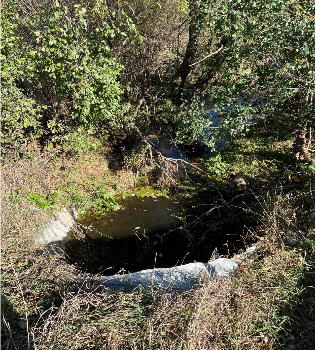
Photo 3 – Downstream side of USH 12 culvert.
