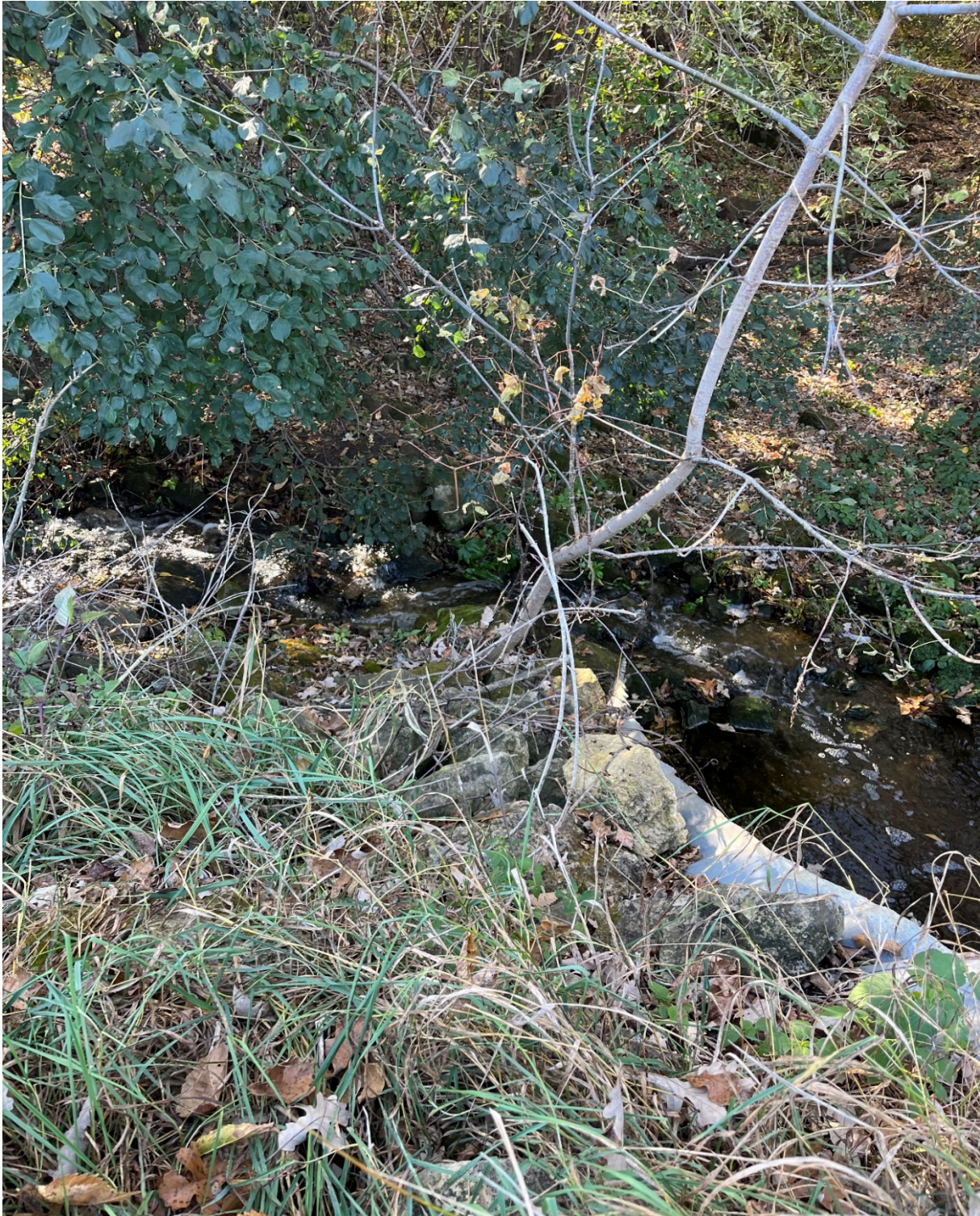
Photo 1 - Effluent discharge on left, before entering culvert under USH 12 and flowing northwest towards Wilson Creek.
