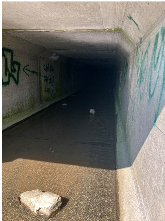
Figure 9. Culvert under Nicholson Avenue, looking west (upstream).
